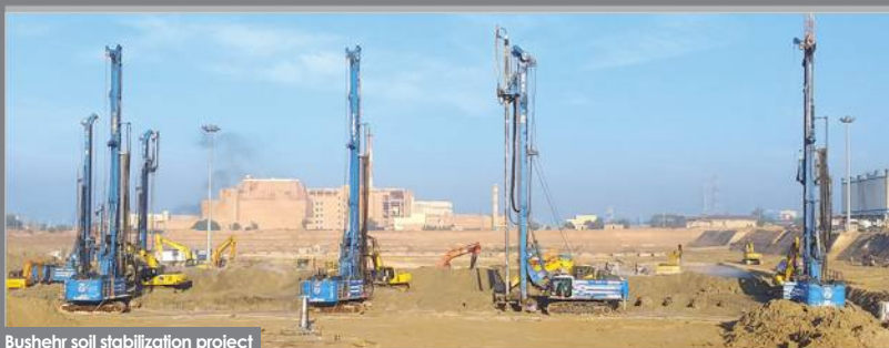
Bushehr soil stabilization project
