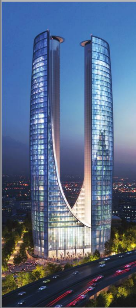
● Saman Faraz Administrative towers
