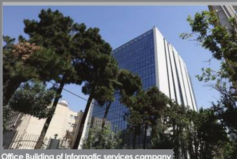
Office Building of Informatic services company
