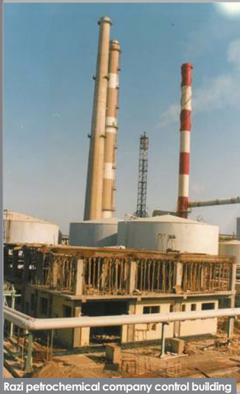
Razi petrochemical company control building
